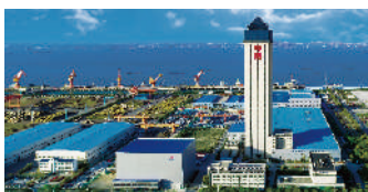
Hengtong Changshu International Marine Industrial Park
