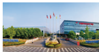
Hengtong Optoelectronic Cable Industrial Park (Qidu, Suzhou)
