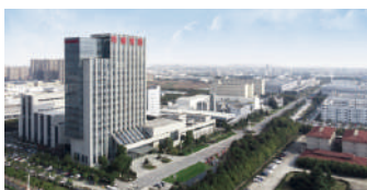
Hengtong Optical Communication Technology Park (Wujiang, Suzhou)
